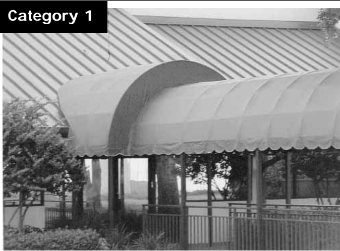
Carports, Canopies and Walkways Winner: West Coast Awning of Clearwater
